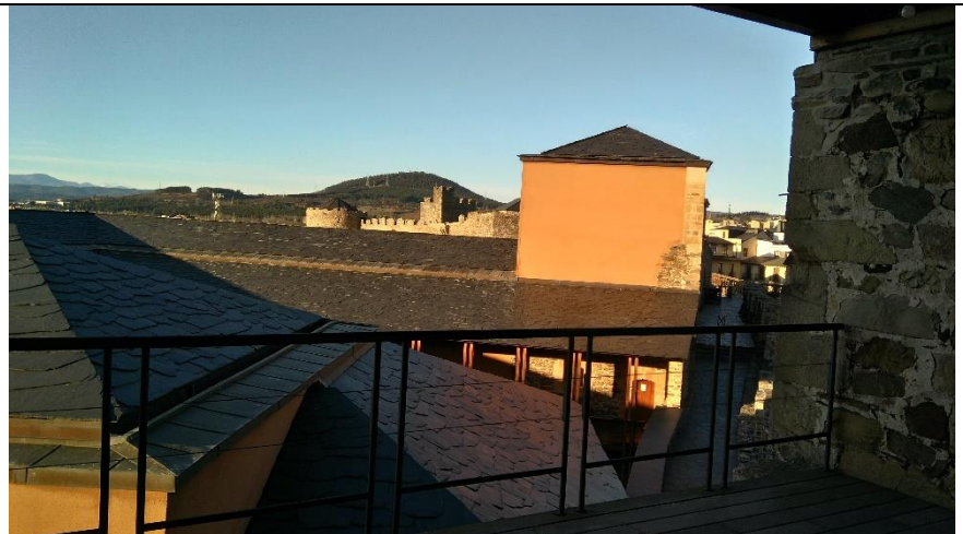
Cabrera Tower. Level 5. View towards the interior.
